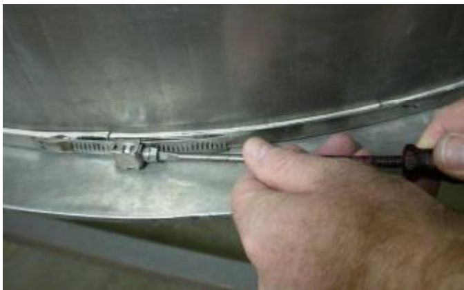
Installation of rubber backed edgeband.
